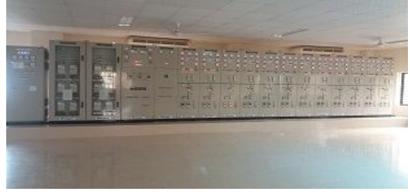
Munshiganj 33 KV Switching Station with 12 Nos 33 KV Circuit Breaker
