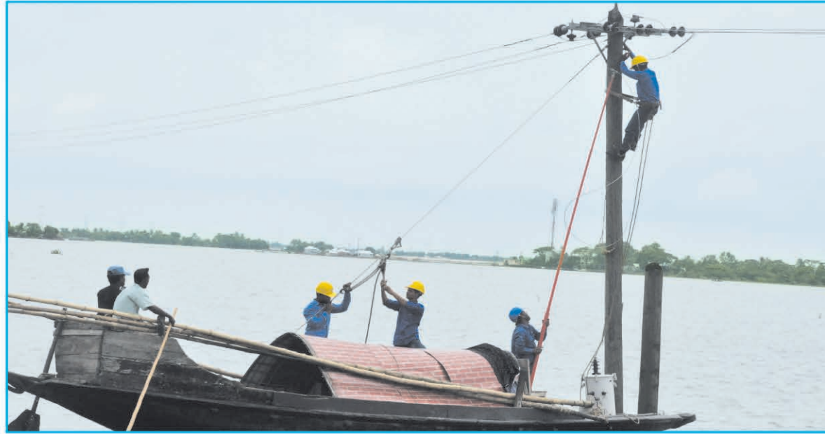
Electrification in haor area in Kishoreganj
